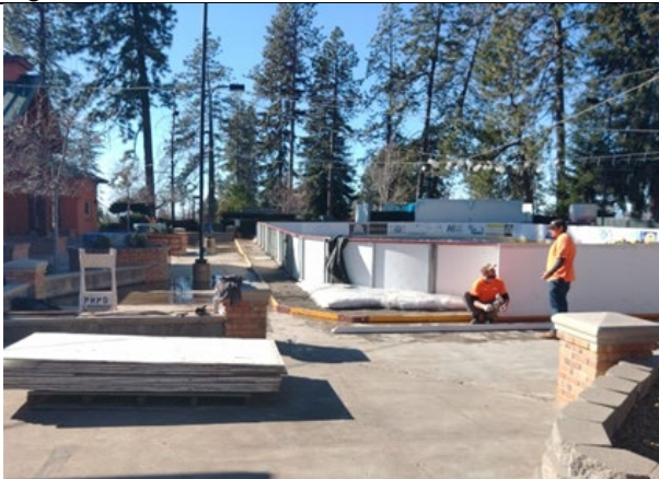
Figure 3. Crew dismantling the Ice Rink.
