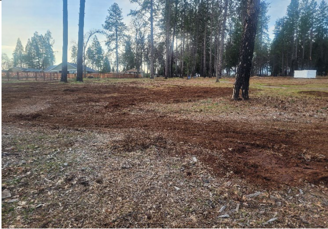
Figure 7. All tree stump removal has been completed at Bille Park.
