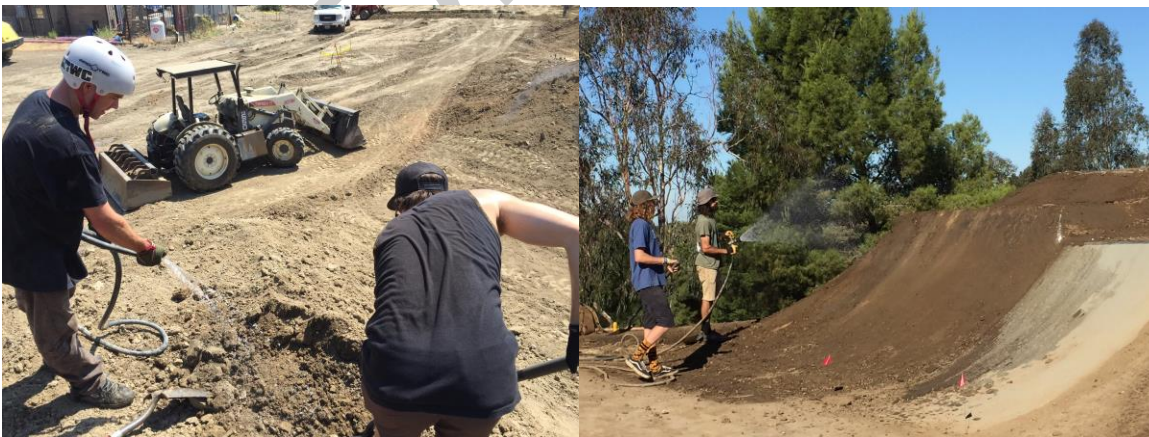
Workers processing materials mixing soil and water together and continue to moisture condition throughout the process to ensure good compaction.
