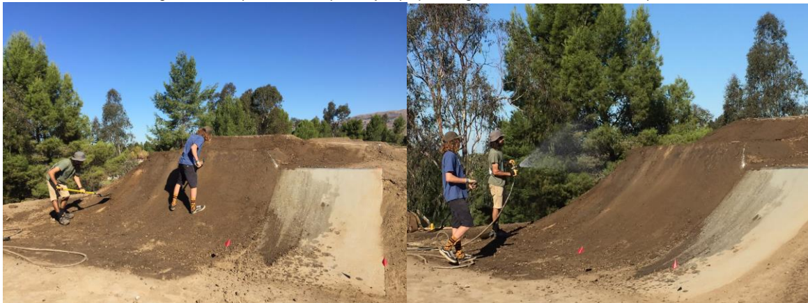
Continue to moisture condition, soil condition, shape and compact throughout the process.
