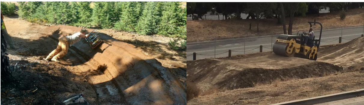
Compacting a berm turn with a vibrating plate compactor. Compacting the large dual slalom features with a roller compactor.
