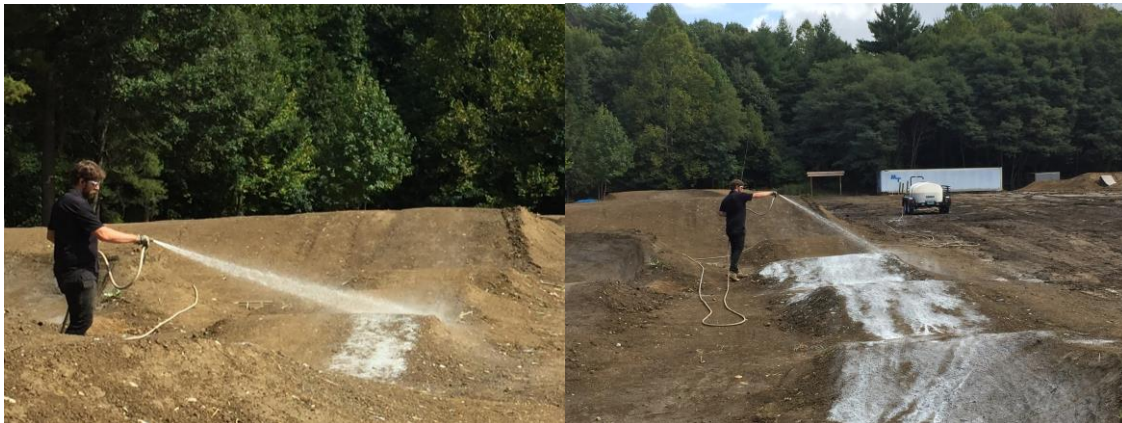
Applying soil stabilizer at the beginning of the season to extended the functional of a pump track.
