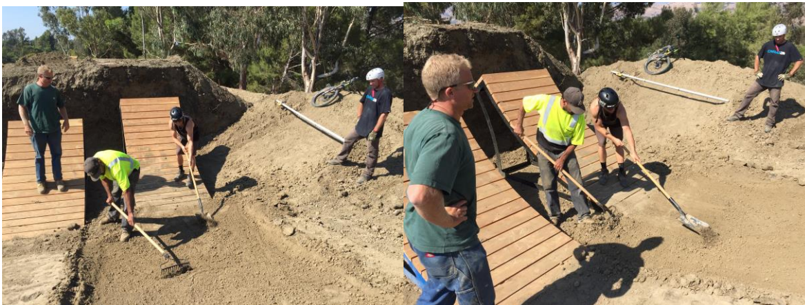
Condition soil with rake or shovel, chop up clods, then smooth, shape and compact.
