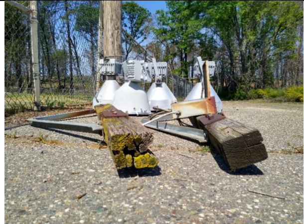
Figure 6. Old pole components
