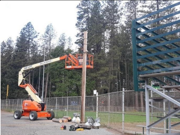
Figure 5. Pole removal project
