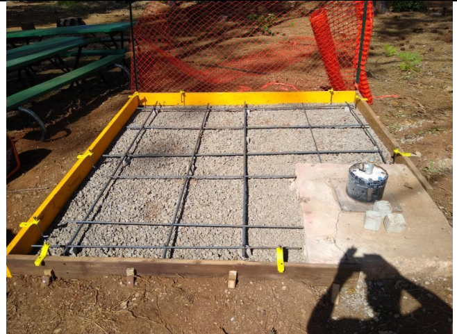
Figure 14. New well pad prep
