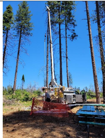
Figure 16. Well being drilled
