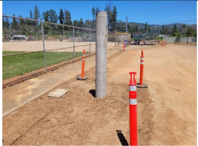
Figure 8. First metal pole base installed
