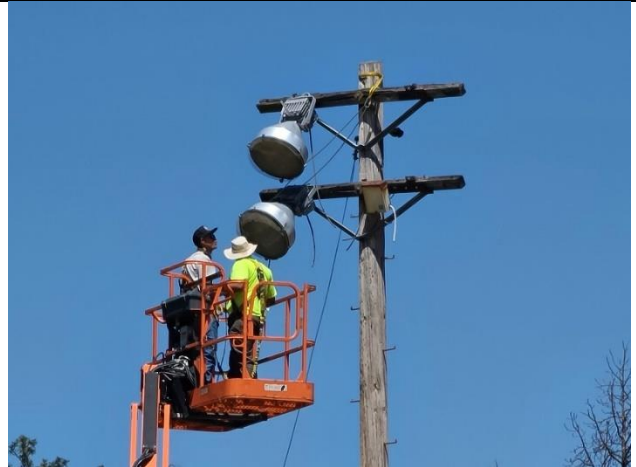
Figure 4. Workers deconstructing old light poles
