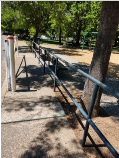
Figure 9. Railing at Aquatic Park before repainting
