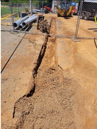
Figure 7. Trenching for undergrounding electrical for new light poles
