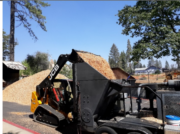
Figure 3. Loading wood chips into the spraying machine.
