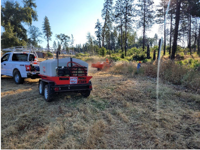
Figure 1. The new shop property during clearing.
