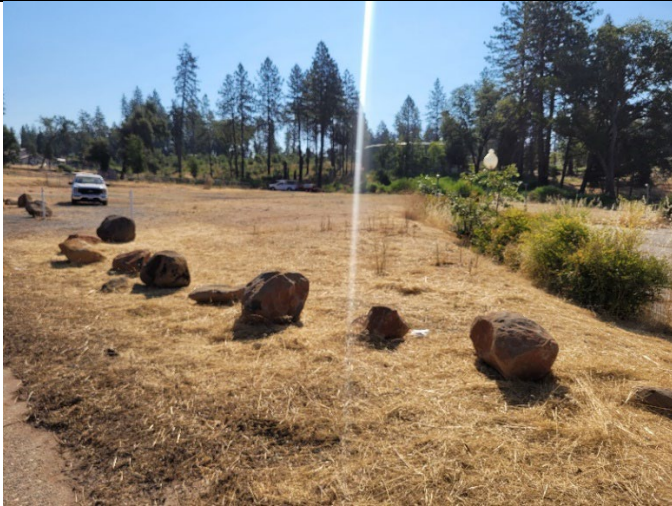
Figure 3. The new shop property after clearing.
