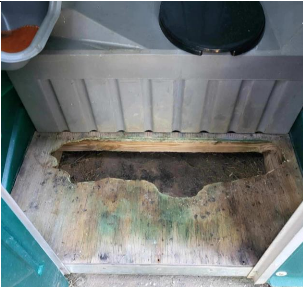
Figure 9. Port-a-Potty before new flooring was installed.
