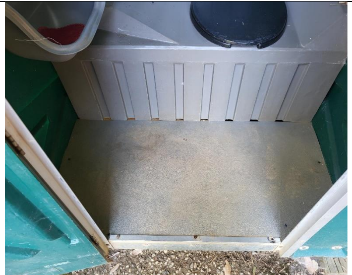
Figure 10. Port- a- Potty after the new flooring was installed.
