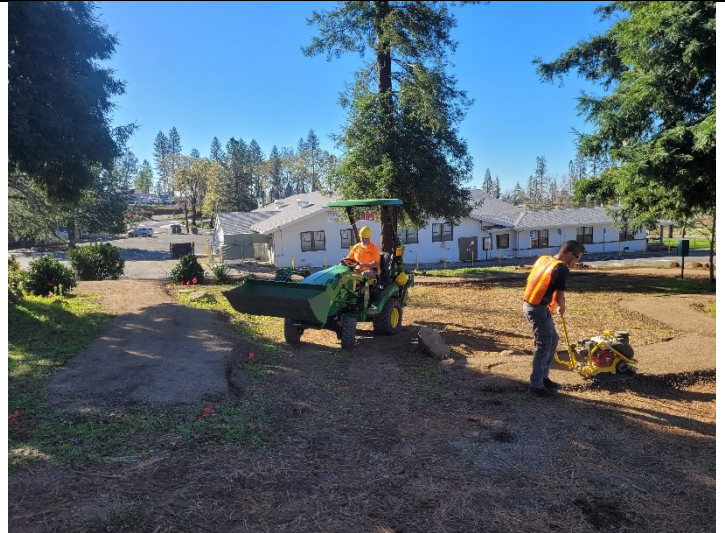
Figure 8. The maintenance crew clearing an area for the new walking path.
