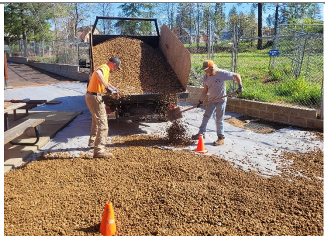
Figure 6. The maintenance crew removed the bark at the TARC and replaced it with rock.
