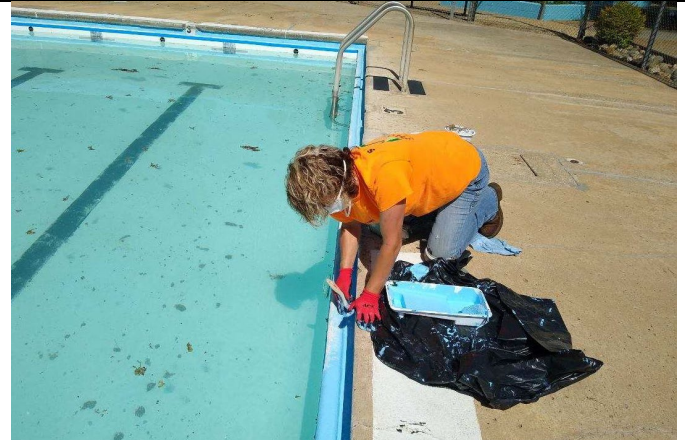
Figure 4. Maintenance employee painting the gutters at the pool.
