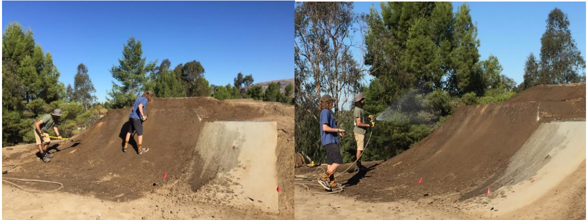
Continue to moisture condition, soil condition, shape and compact throughout the process.
