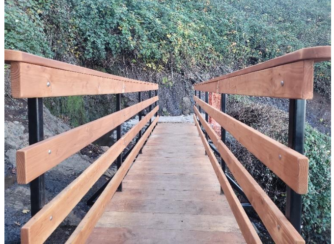
Figure 2. The newly built bridge at the grotto.
