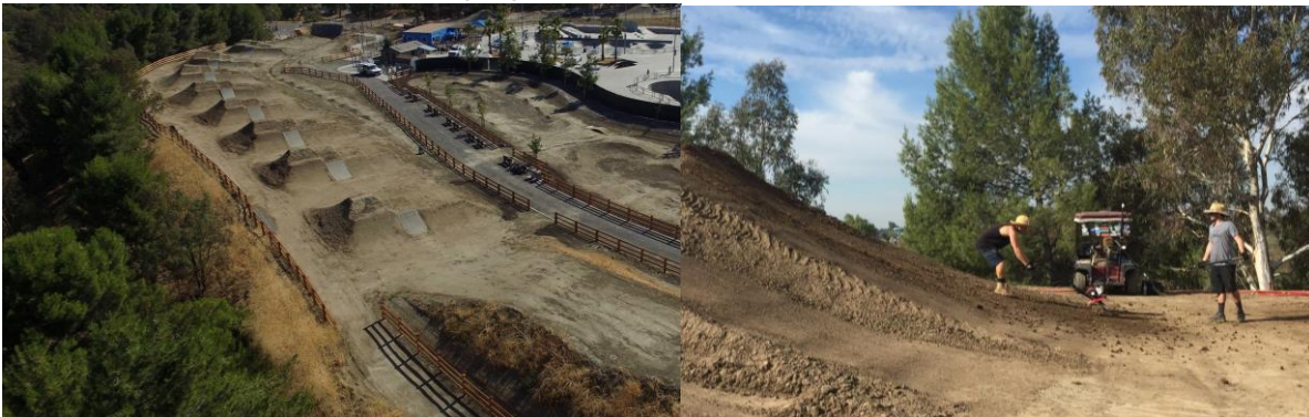
Finished jump set. Using a tiller to condition soil and fine tune landing.
