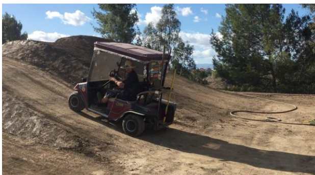
Using a push broom to smooth out the jump lip and prep for final compaction. Final compaction with golf cart.
