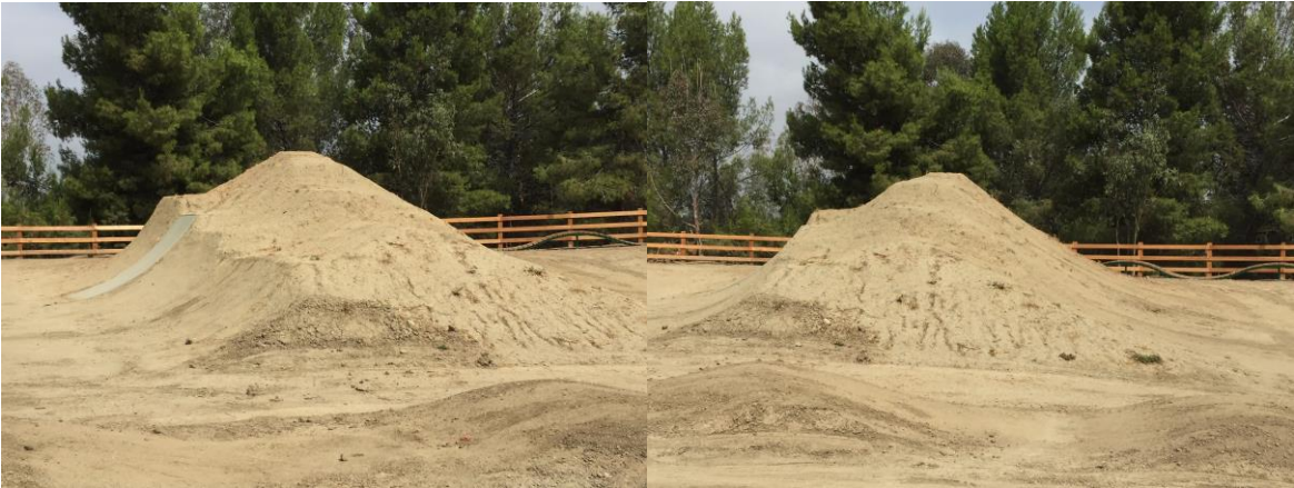
Final shape jump set with kicker lip on the front end and a lander transition on the back end.
