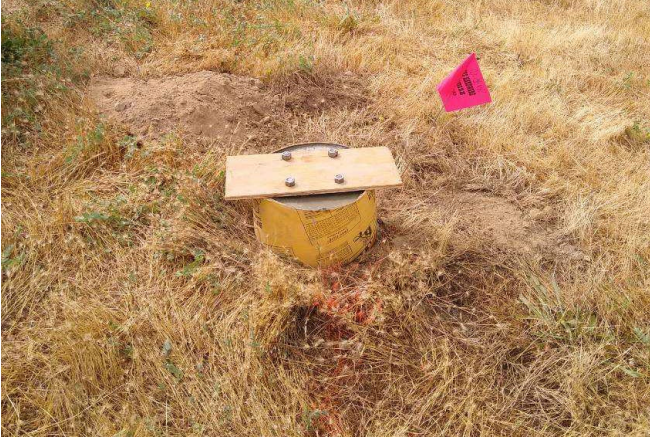
Figure 1. PRPD staff starting the pedestal installation for plant signs.
