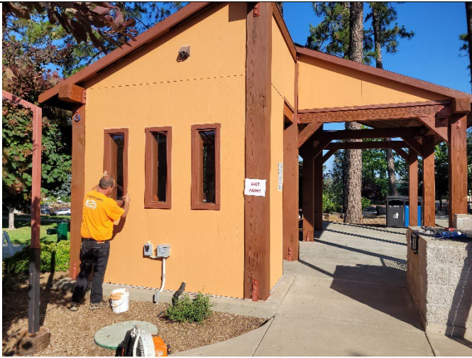
Figure 5. The BBQ area after it was repainted and stained.
