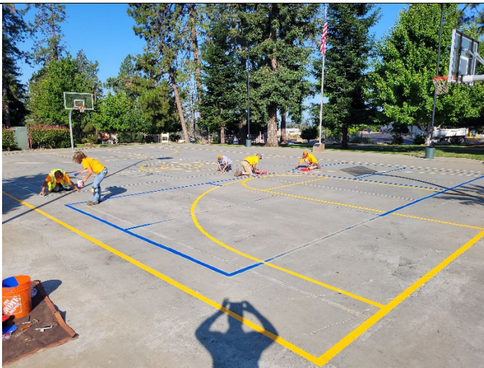
Figure 7. During the paint job.
