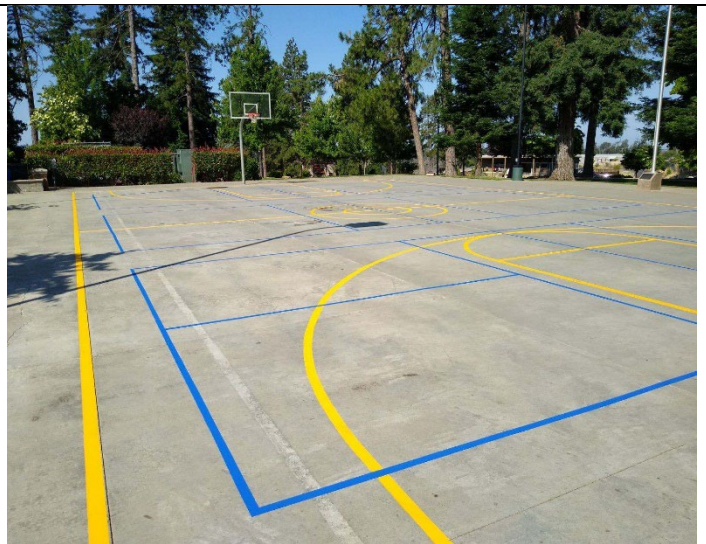
Figure 8. After the completion on the paint job.
