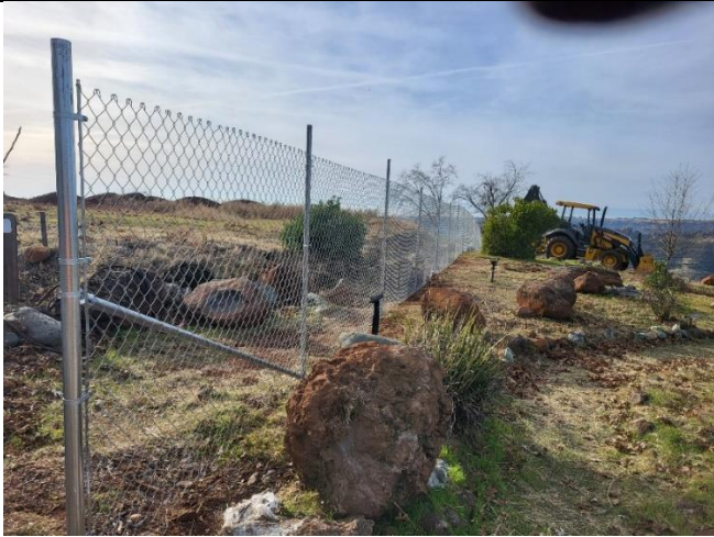
Figure 5. The completed fencing at the Forty Oaks property.
