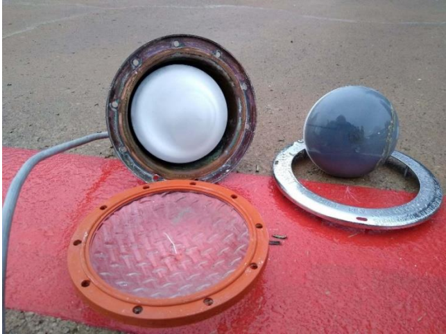
Figure 1. Maintenance, changing out the gaskets and bulbs on the pool lights.
