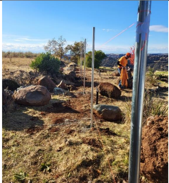
Figure 4. Fencing going up at the Forty Oaks property.
