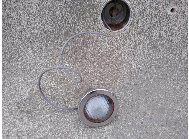
Figure 2. Maintenance, changing out the gaskets and bulbs on the pool lights.
