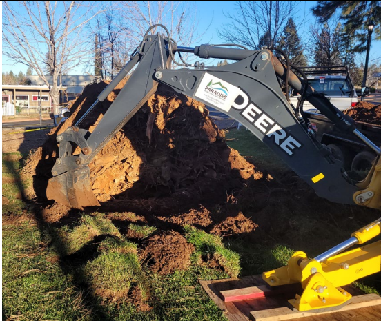
Figure 2. Maintenance crew working on getting the stump back into the ground.
