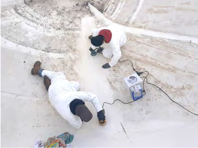
Figure 1. Prepping for epoxy paint application
