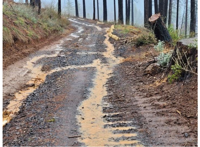
Figure 2. Erosion Control on Merchant Bar Road
