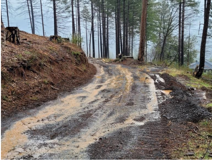
Figure 1. Erosion Control on Merchant Bar Road.
