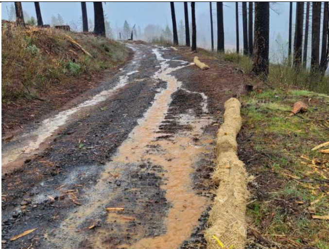
Figure 3. Side barriers added on Merchant Bar Road
