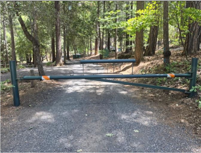
Figure 9. Repaired gates at Paradise Lake.
