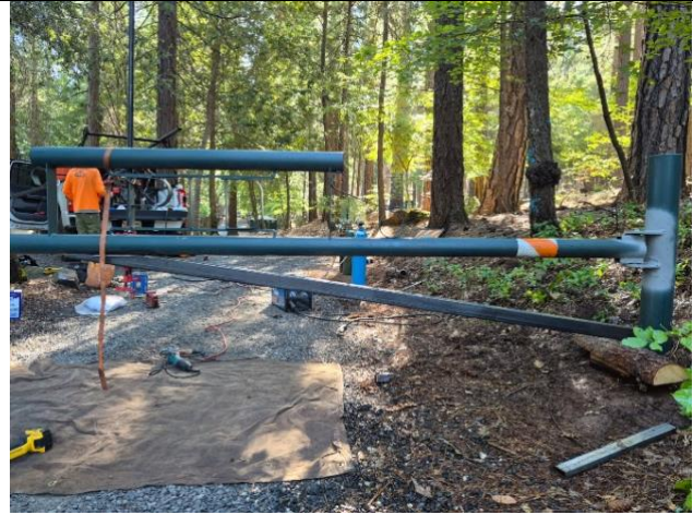
Figure 8. Repaired gates at Paradise Lake.
