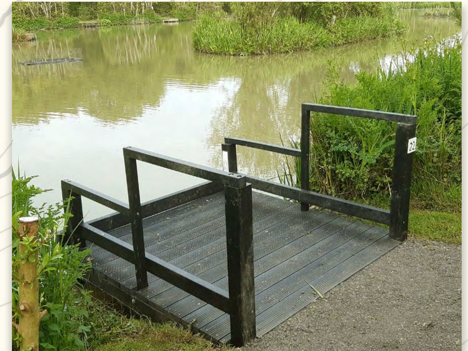
ADA fishing platform with railing
