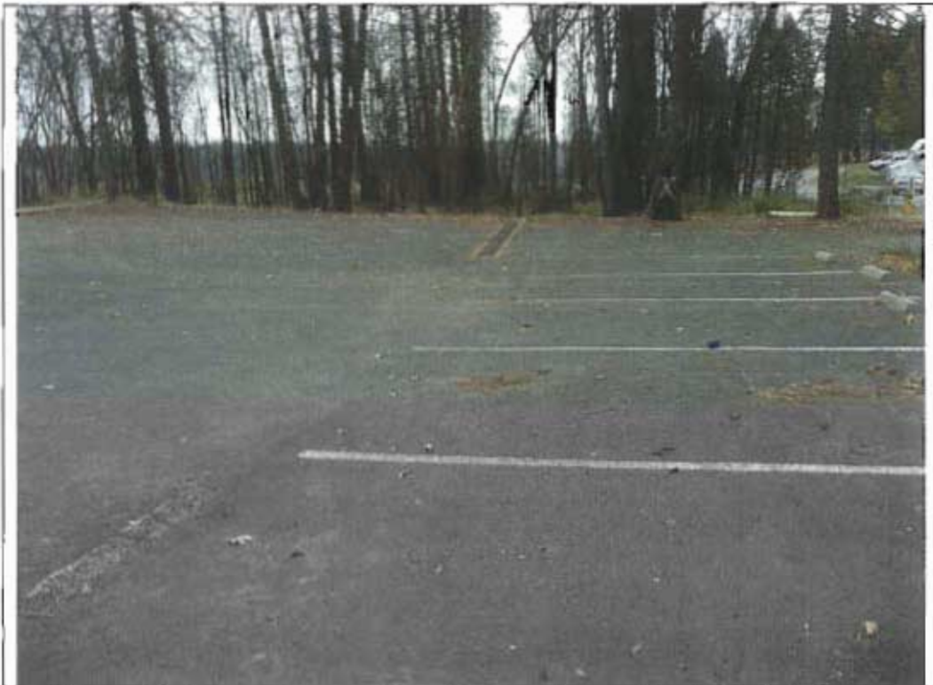
Looking south from western portion of lot showing parking lot and drainage. (297)
